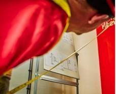
> 1.3 Finally measure the diagonals. Once you're satisfied that all the measurements are acceptable proceed to fitting the sub-cill (Step 2).
