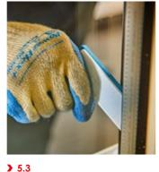
Pack glass down the sides (two each side - one at the top and bottom of each stile and not central).
