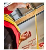
> 1.2 Next, measure the vertical dimensions at each end of the opening and again in the centre.
