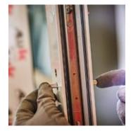
> 4.3 Fit lock spindle and handles (if not already fitted).
