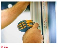
Insert perimeter fixings and pack frame (ideally use u-shaped packs). Be careful not to over tighten as this may deform the frame. Check again for plumb, level and squareness.
