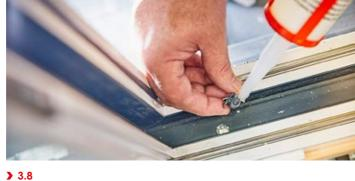
Insert the drainage pieces into the central channel. These should be sealed with a small amount of sealant before insertion and lightly tapped home to ensure they're seated correctly.
