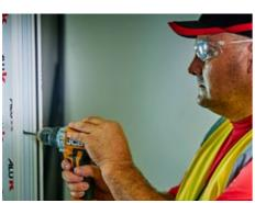
> 3.5 Don't forget, fixing centres should be 100 - 150mm in from each end and a maximum of 600mm thereafter. Drill and counter-bore pilot holes through the thermal break.
