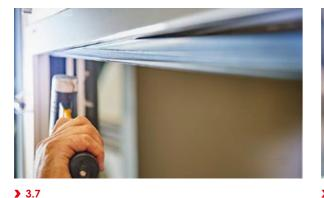
When you're completely satisfied the frame is fitted plumb, level and square, replace the plastic channel around the frame.
