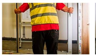
> 4.1 Lift first door leaf into position and seat on track. Don't forget, if working from the outside this will be the internal leaf. Operate the door a few times to
