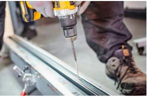
Give it a final level check and adjust if necessary. Once you're happy the sub-cill is level it's time to fix it to the cill.
