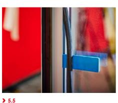
Fit the wedge gasket, ensuring the gasket isn't stretched and is cut oversize by 10mm per meter. Remember to force into the corners first and then loop from the centre towards the corners.
