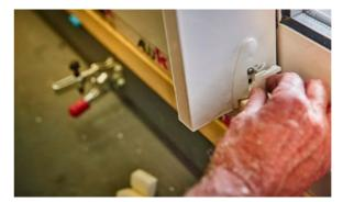
> 6.1 Seal the frame to the substrate using a proprietary sealant.
