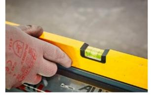
> 2.3 Recheck and adjust the packers as required and bed on a suitable material. Check for bowing in the cill by using a laser level or spirit level (or old school builder's string line).
